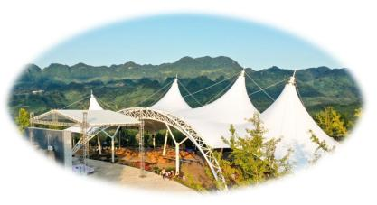
Membrane structure is a structural system that combines architecture and structure. It uses high-strength flexible film materials and auxiliary structures to generate a certain pre-tensioning stress inside and form a certain spatial shape under stress control as a covering structure. or the main body of a building, and has sufficient rigidity to resist the action of external loads of a narrow type of structure.
