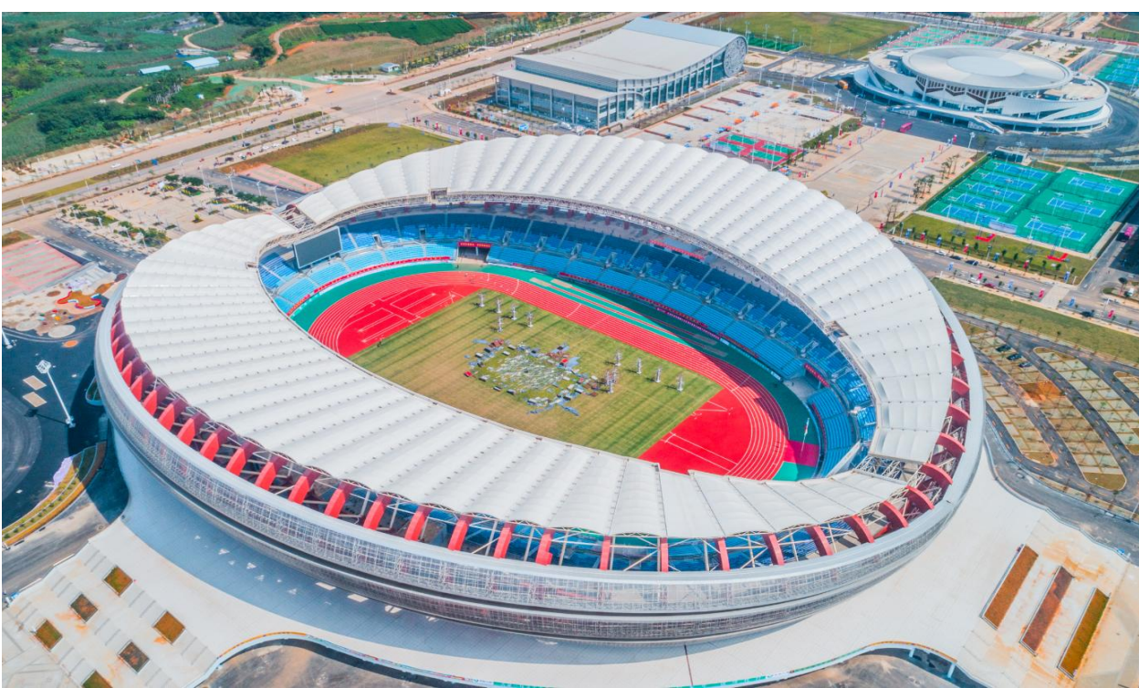
Membrane structure of the main stadium of Chongzuo Sports Center
